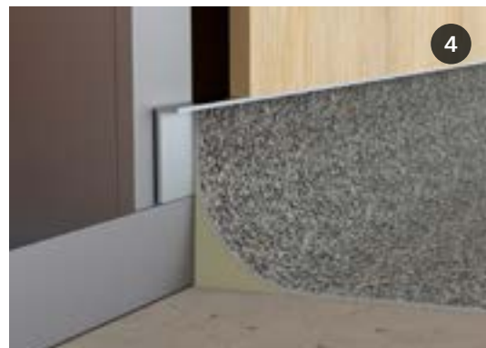
Raised vinyl floor
